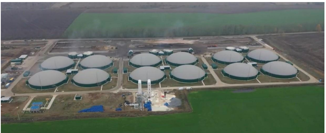
Fig. 2. Biogas complex of MHP "Oril-Leader"
