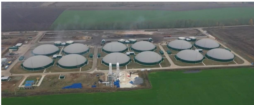
Fig. 2. Biogas complex of MHP "Oril-Leader"
